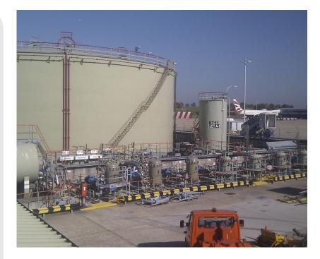
This client is the busiest single-runway airport in the world. With more than 660 aircraft movements daily, the efficiency of all aircraft fuelling systems is critical. The airports storage and hydrant company was faced with the critical challenge of maintaining a constant hydrant pressure of 7.5 to 9 bar. The pressure of the fuelling pumps, however, is directly affected by the number of aircraft being fuelled simultaneously. If the pressure in the fuelling pumps drops, flights are delayed.
